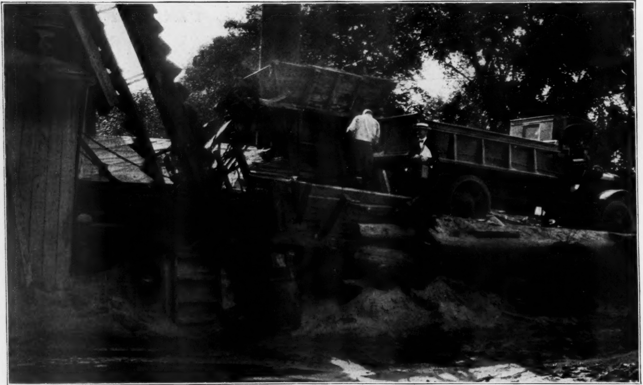
Truck Unloading at Grizzly
